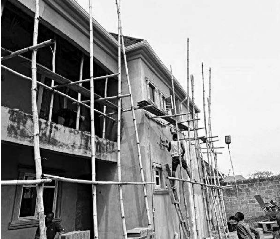
•A house being screed with locally produced material.
