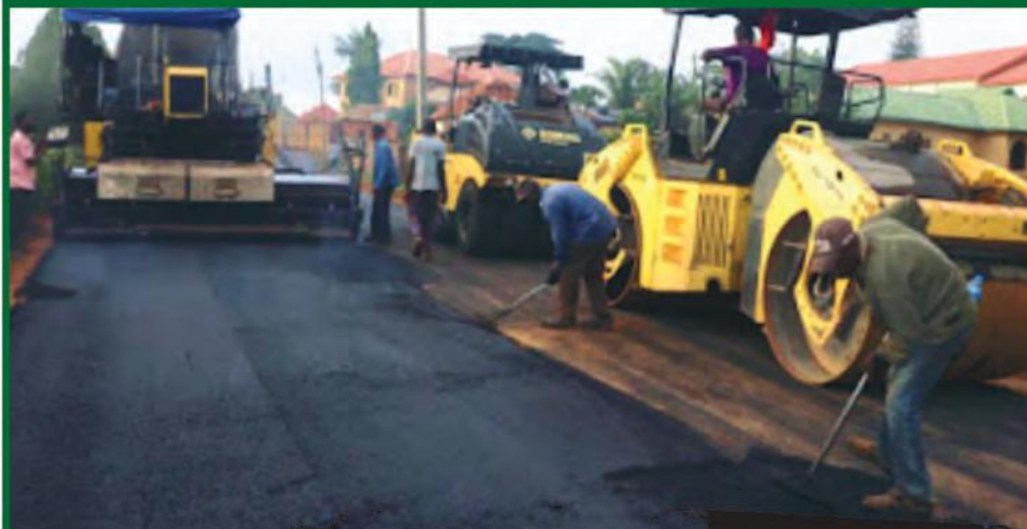
Angwan Rukuba-Bauchi Road Junction
