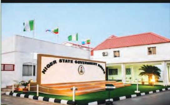
Ongoing face lift of the Niger State Government House.
