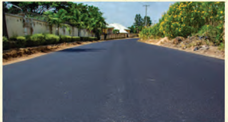
Liberty Boulevard (Millionaires Quarters)
