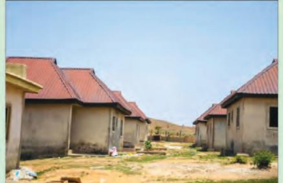
Ongoing construction of 300 units housing estate.
