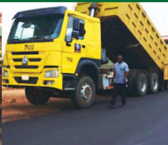
Building Materials-NOUN-Sabon Barki-Bukuru Lowcost Road Network
