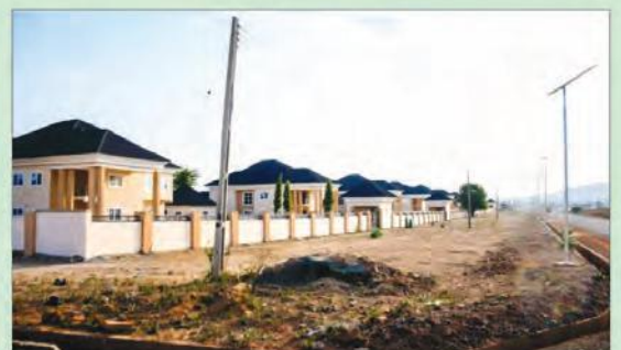
Ongoing remodeling of 3 arms zone
