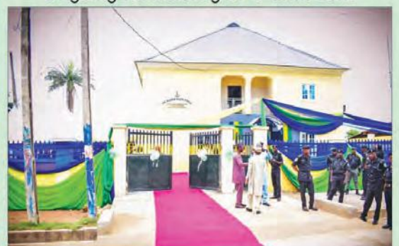
Constructed and commissioned demolished Chanchaga Divisional Police Station
