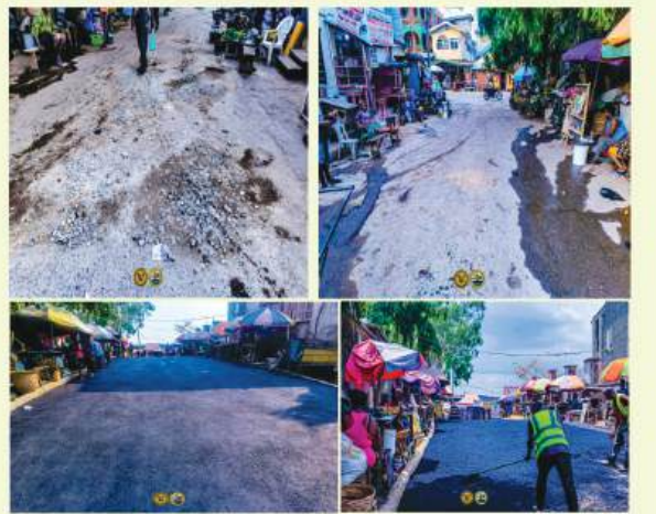
CONSTRUCTION OF DADA AGA STREET ERUNKAN MILE 17
