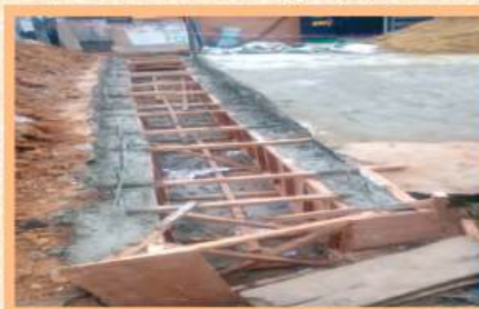
•Construction of drainages
